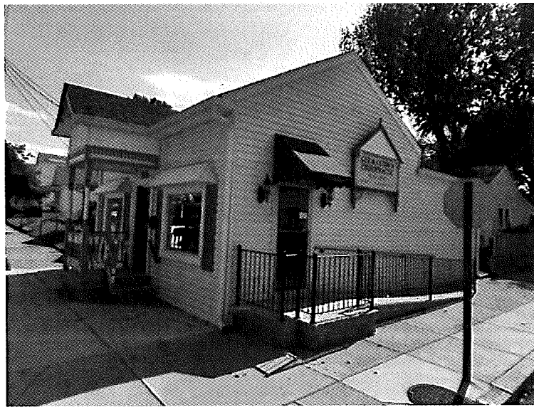
The building at 1100 Milton St. prior to the fire earlier this year. | Courtesy of Jefferson County PVA
