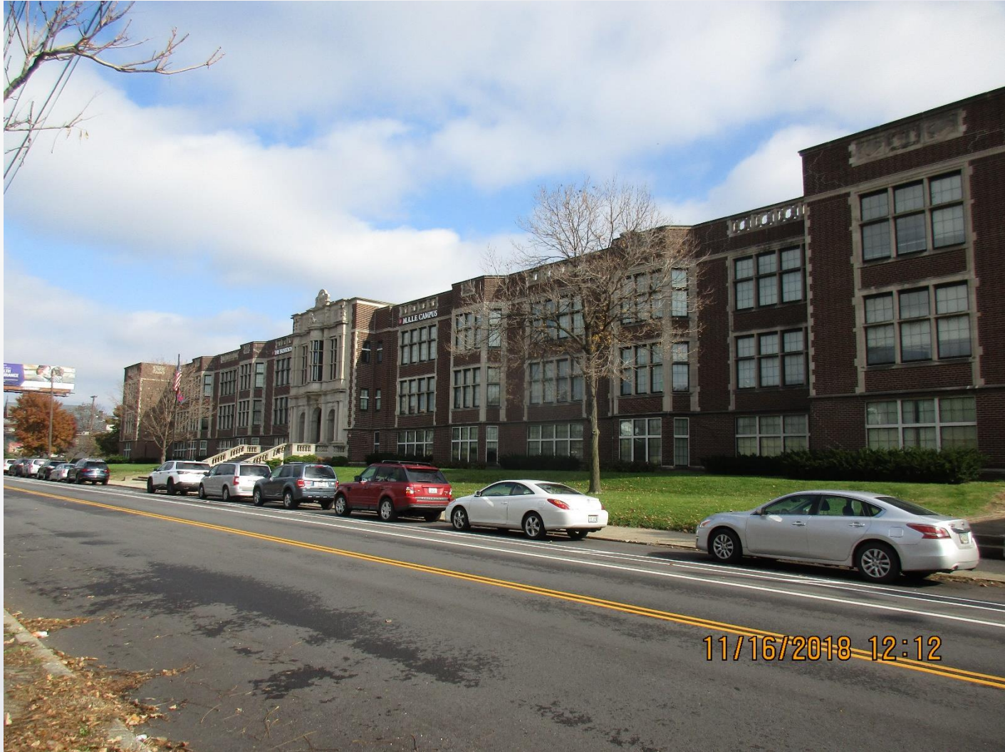
Facade South to North
