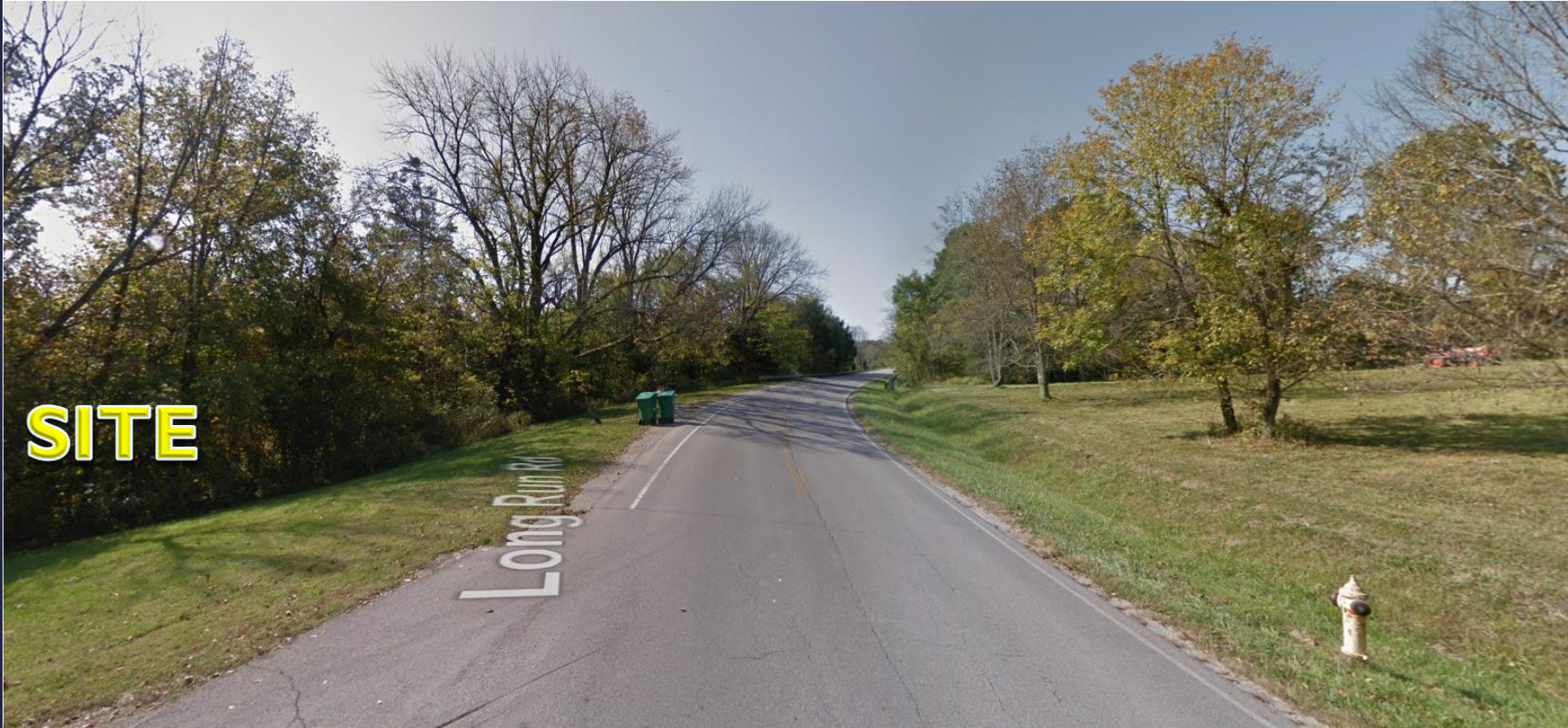
View of Long Run Road at Old Stage Coach Road, looking south. Site is to the left.
