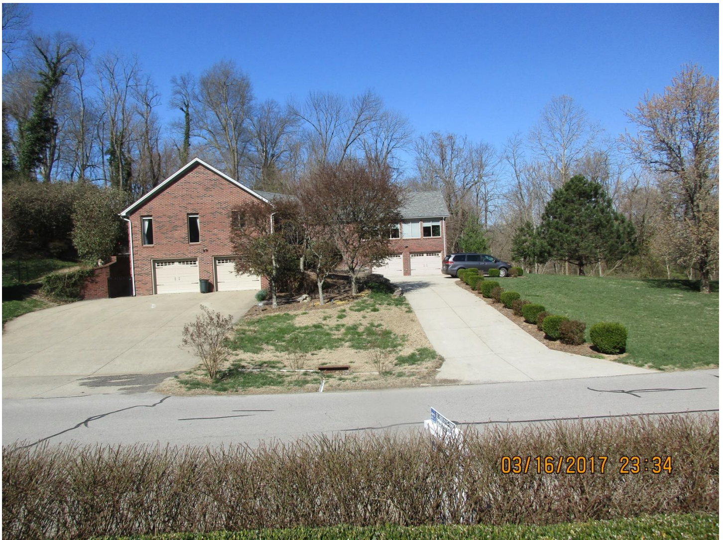
The house across Twin Hill Road.
