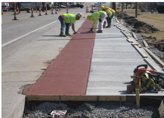
Sample streetscape under construction
