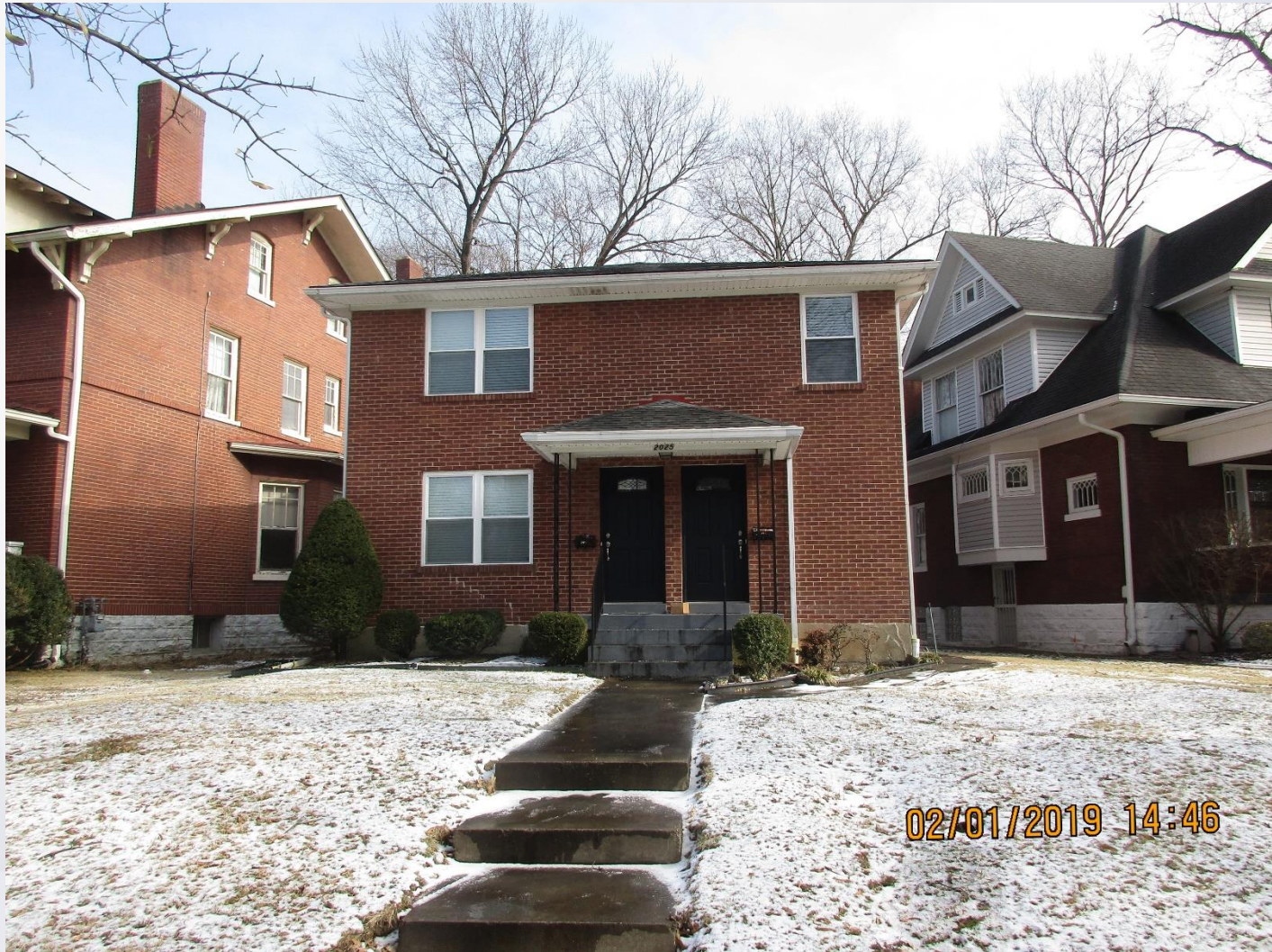
Adjoining to North
