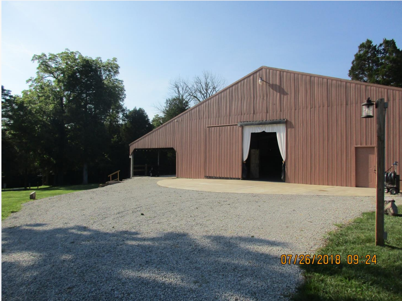
Concrete Pad at Barn Front
