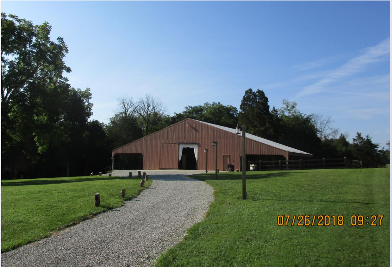
Gravel Drive to Barn
