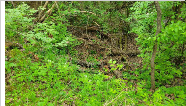
Photo 33: View of "bowl shaped" slope failure (Slope Area 13).
