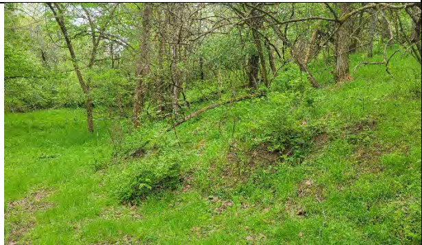
Photo 36: View of soil mounding and minor erosion (Slope Area 13).
