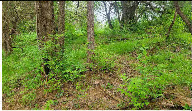
Photo 18: View of soil mounding and minor erosion (Slope Area 9).
