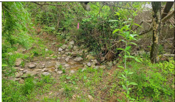
Photo 28: View of culvert and drainage swale (Slope Area 11).
