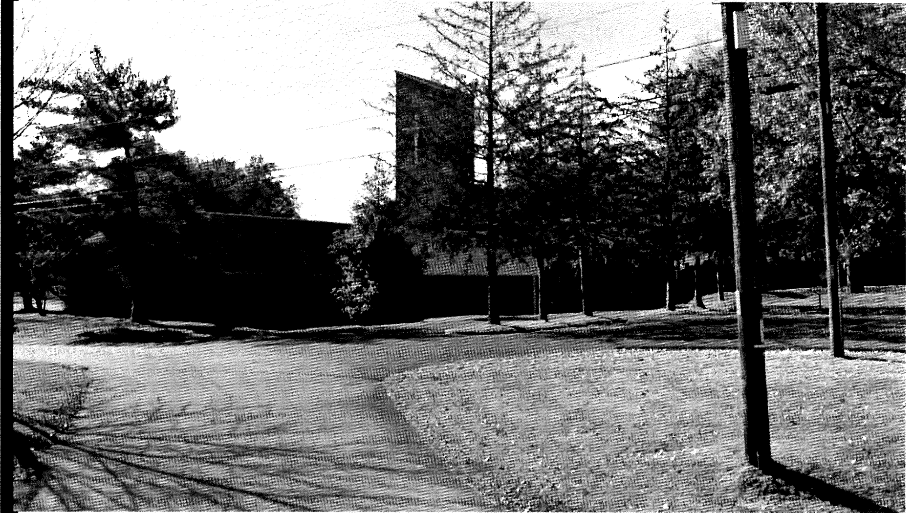
Existing Lifepoint Church, proposed for athletic office and locker room facility.
