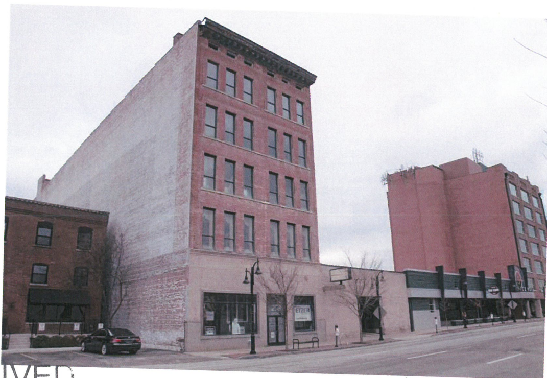
Figure 08 - 209 East Main Street - South and West Facade Facing Northeast
