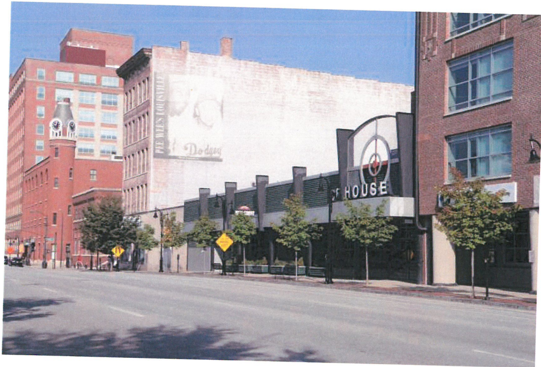
Figure 17 - 209 East Main Street Existing View Facing Northwest On Main Street
