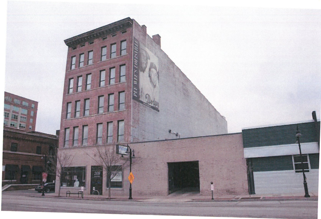
Figure 07 - 209 East Main Street - East and South Facade Facing Northwest
