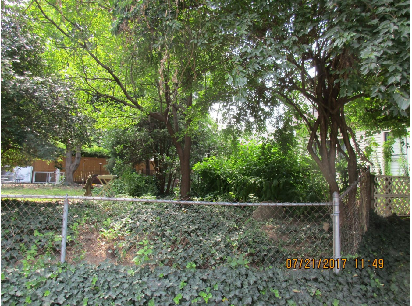
The existing fence to be replaced.
