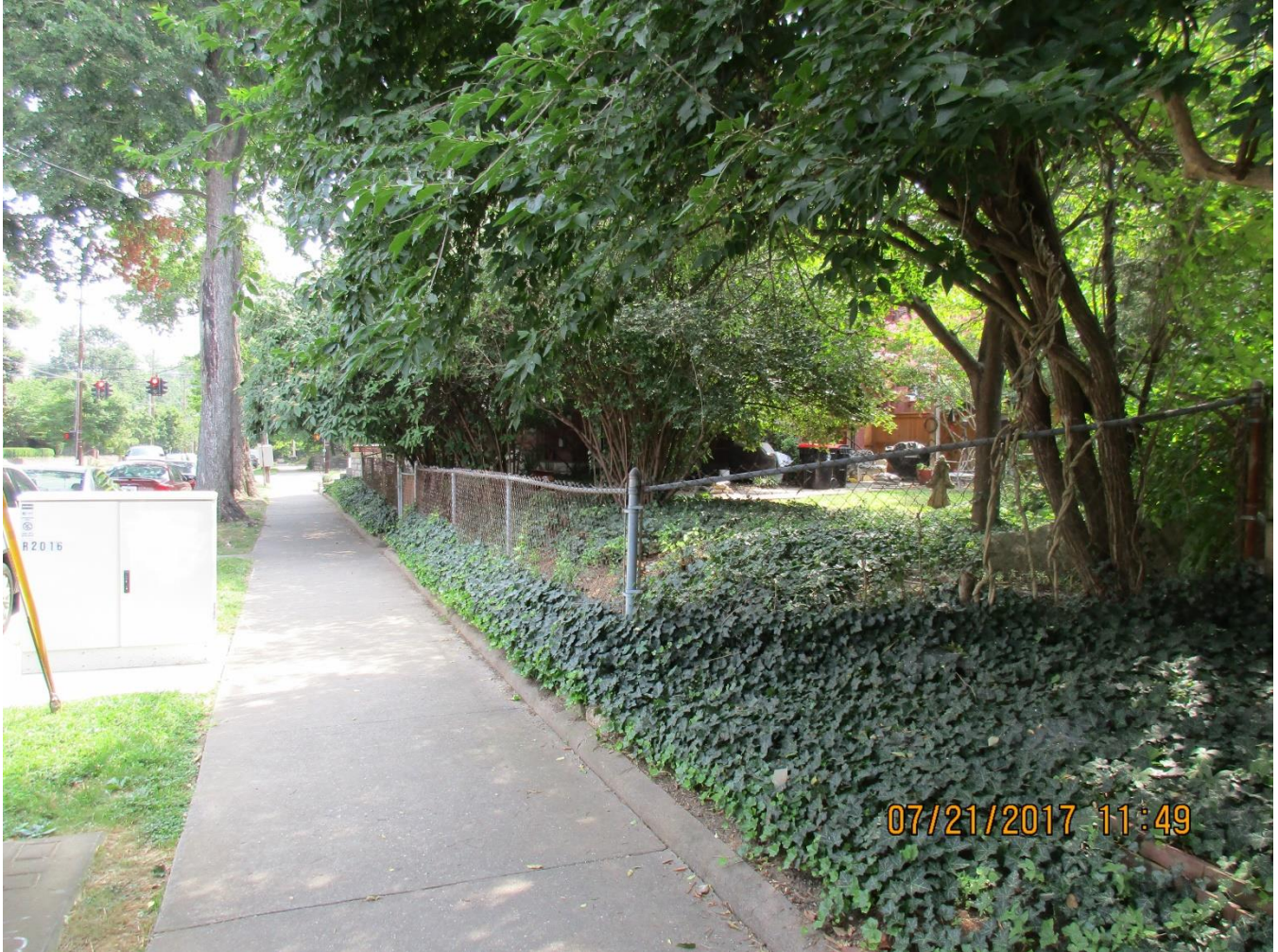
The existing fence to be replaced.
