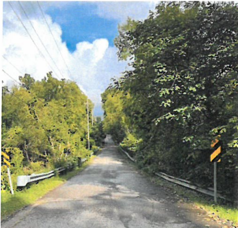
Figure 2.1 - Narrow Laurel Springs Dr bridge marked by hazard signs.
