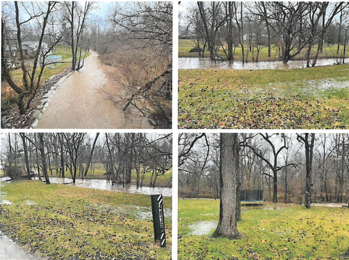
Figure 5.4 - Fern Creek flooding
