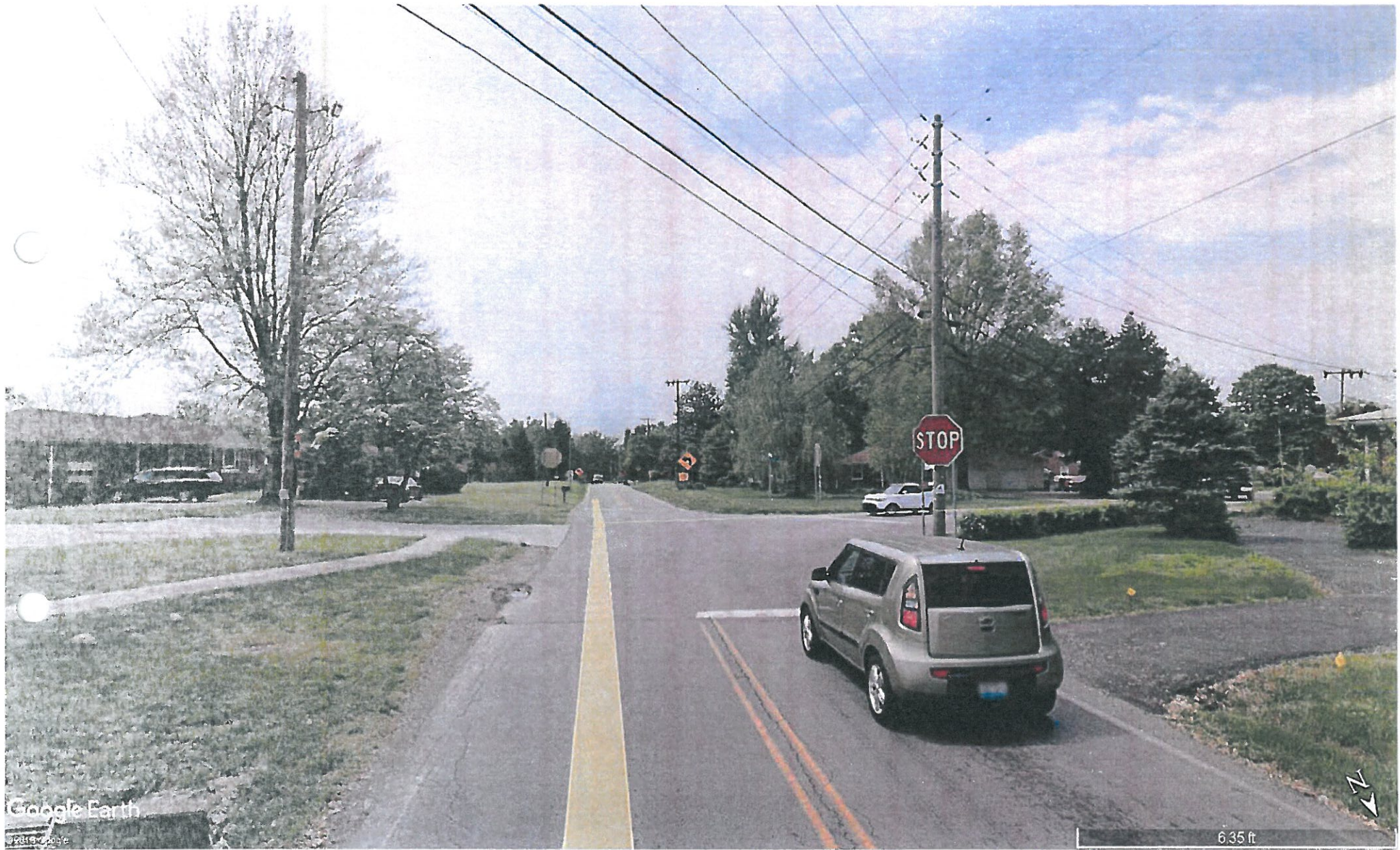
S. on Shepherdsville Rd at 3 way stop with Manslick Rd.
