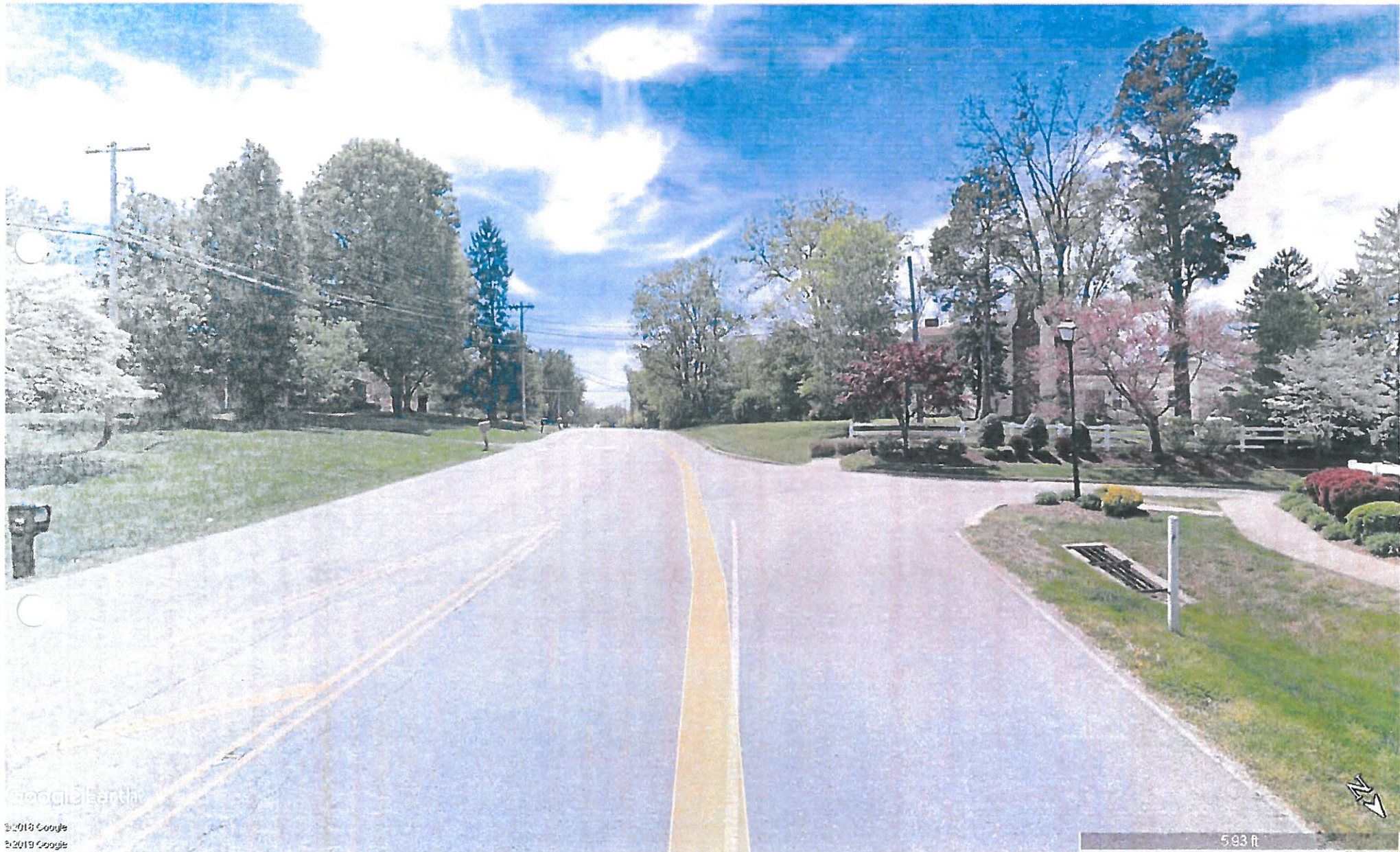
South on Shepherdsville Road at Savannah Springs entrance (on right). Decel lane on right into development and center left turn lane visible in distance.
