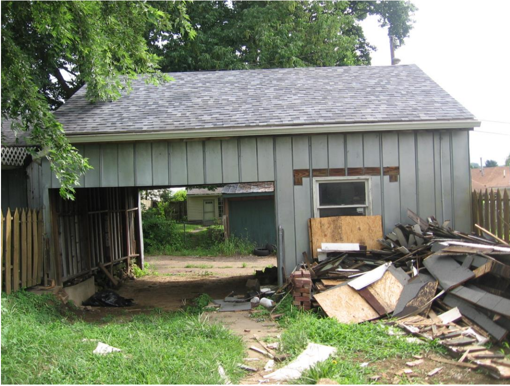
Existing garage at rear of property
