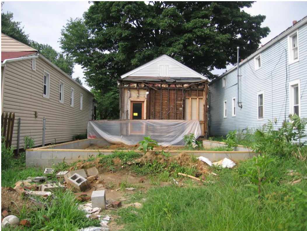
View of rear addition from rear yard
