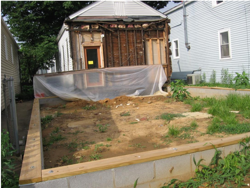
View of rear addition from rear yard
