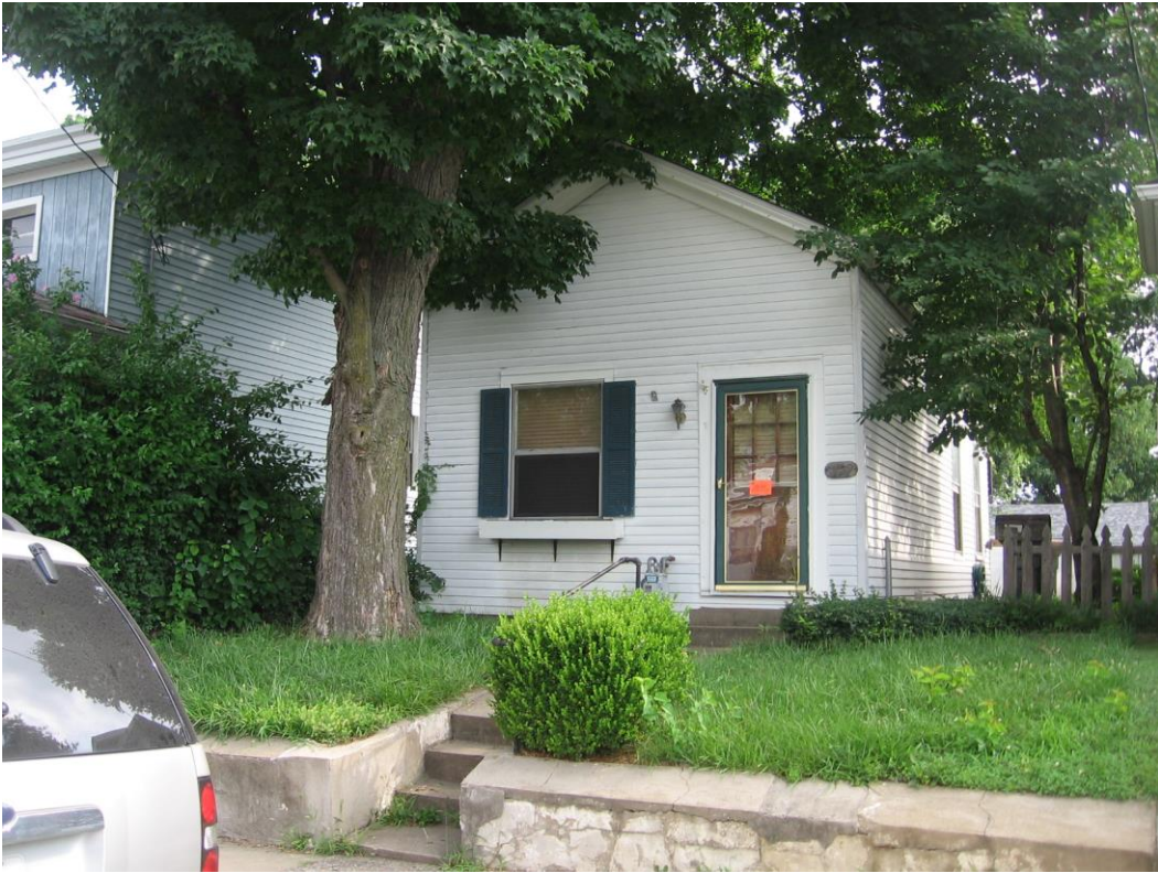
Front of the Existing House
