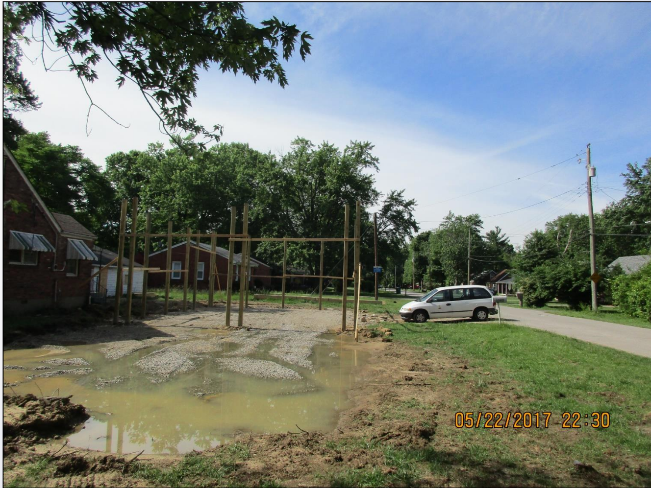
The partially constructed pole barn with sight lines down Daleray Drive
