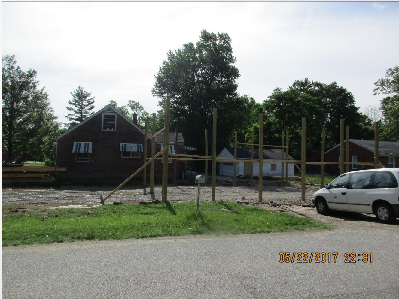
The partially framed pole barn with the residence and existing garage
