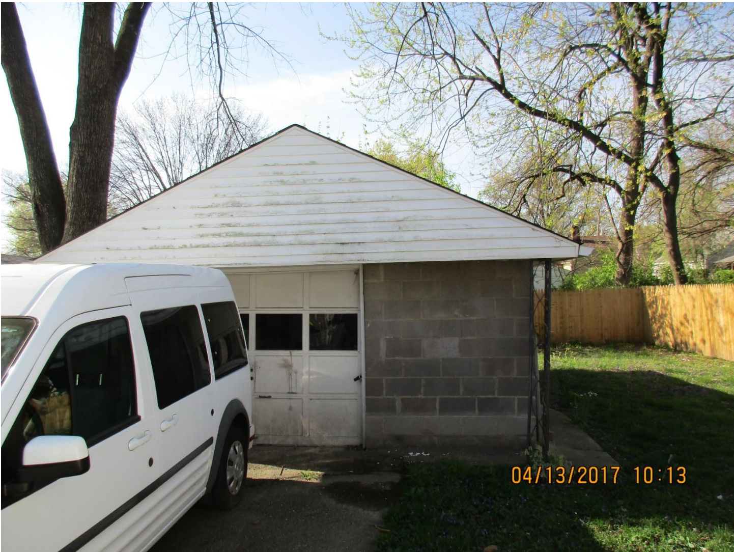
The existing garage.
