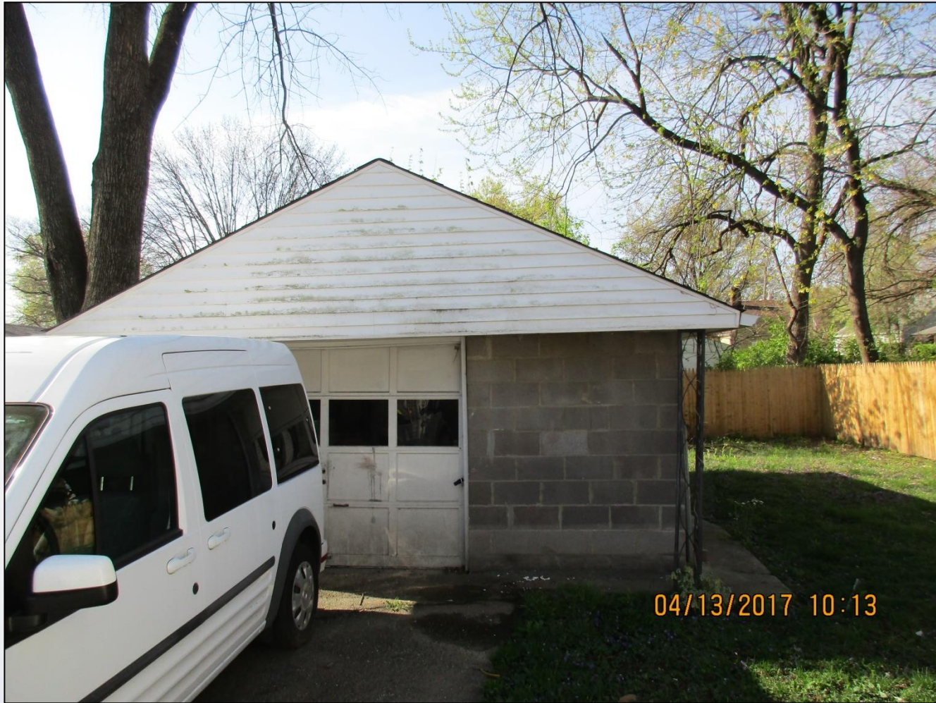
The existing garage.
