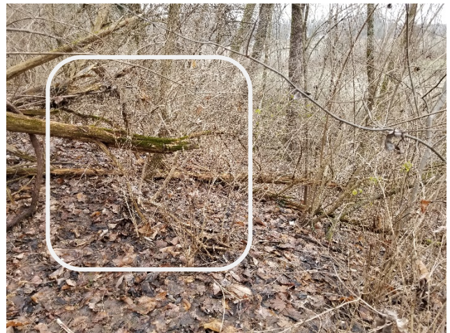
Bent tree and soil mound along the slope at Lot 68
