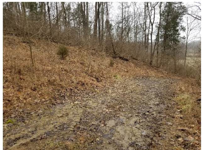
Access road and erosion at Lot 54
