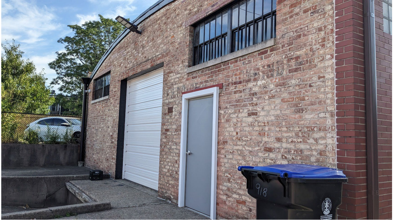
West Rear Façade
