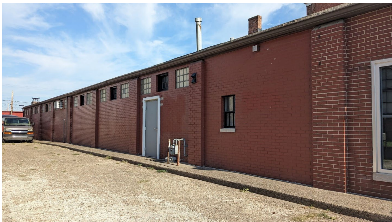
South Side Façade
