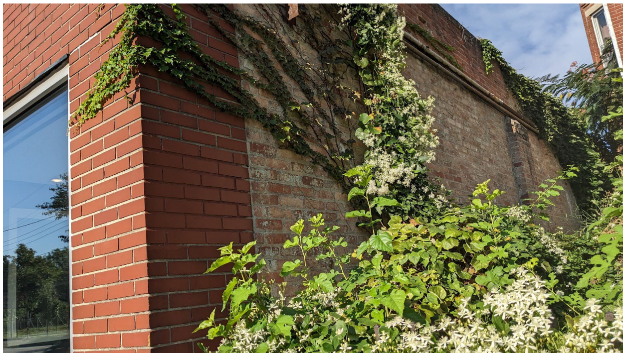
North Side Façade
