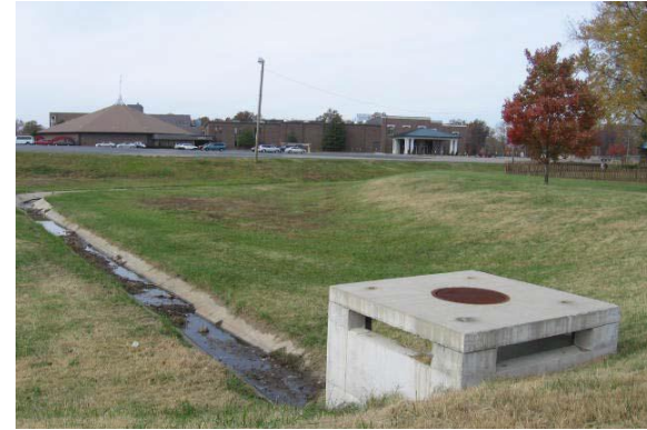
Drainage channel and retention basin
