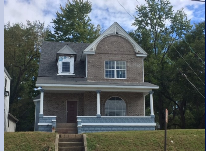
S. 28 th St. after rehab
