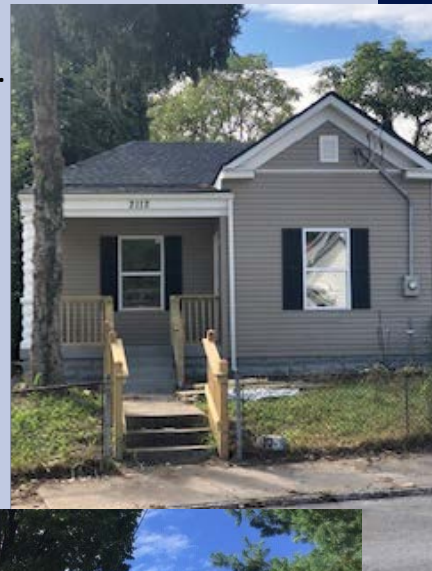
Wilson Ave. after rehab
