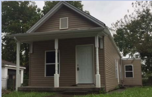
Allen St. after rehab
