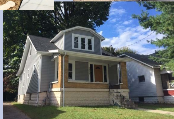
S. 41 st after rehab
