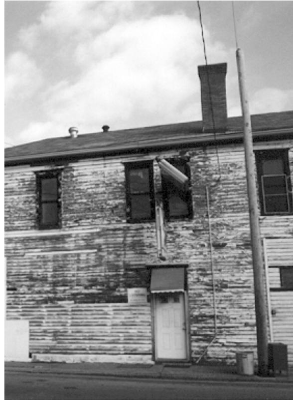
*Coating systems are critical for the preservation of wood features. If left unaddressed, paint failure can lead to serious deterioration.*
