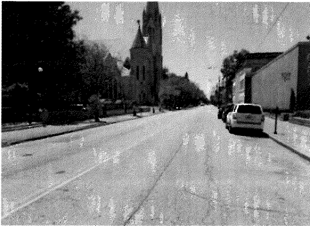
Photo #3: S 4 th St looking south at York St
