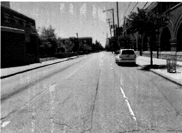
Photo #5: S 4 th St looking south at W Breckenridge St
