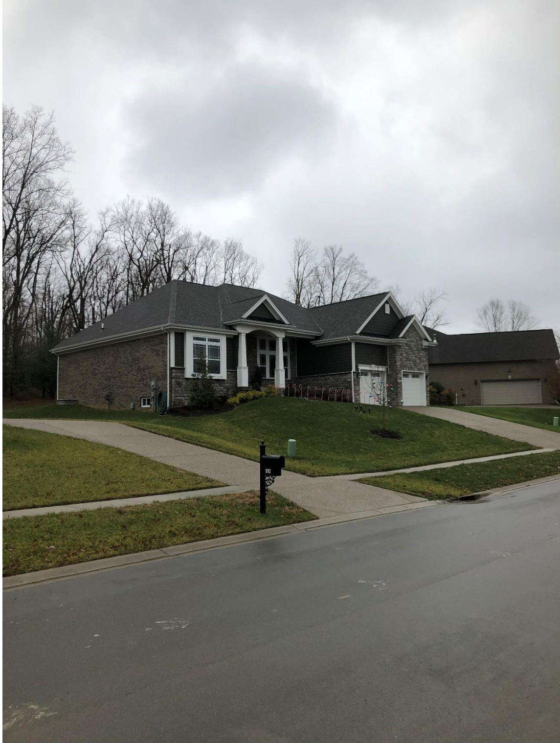
Property to the right of subject property.
