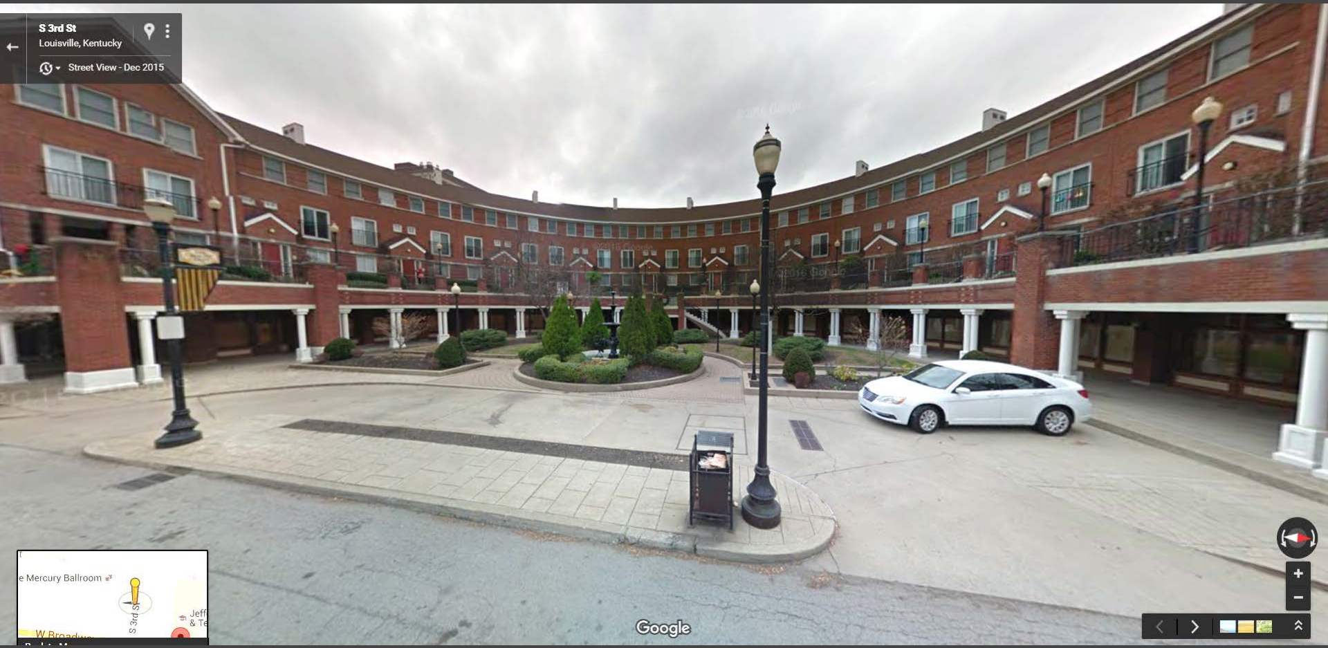
View of Crescent Center (west building) looking west.
