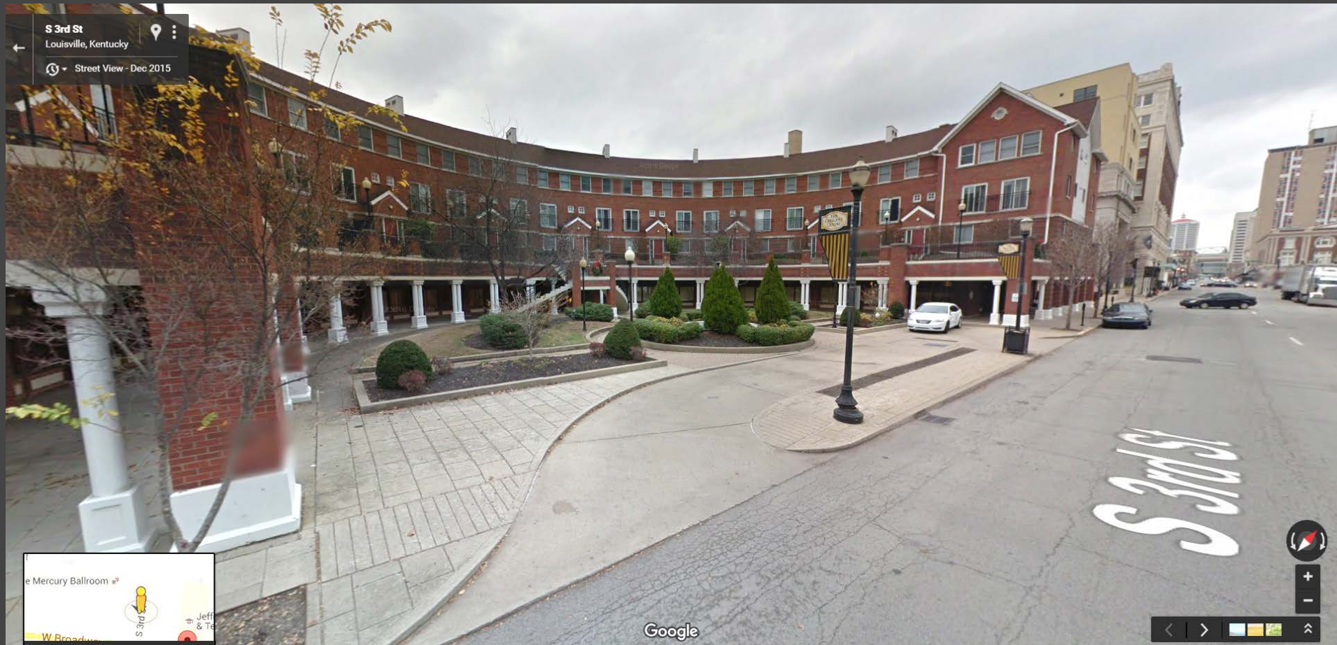
View of Crescent Center (east building) looking south towards Broadway.
