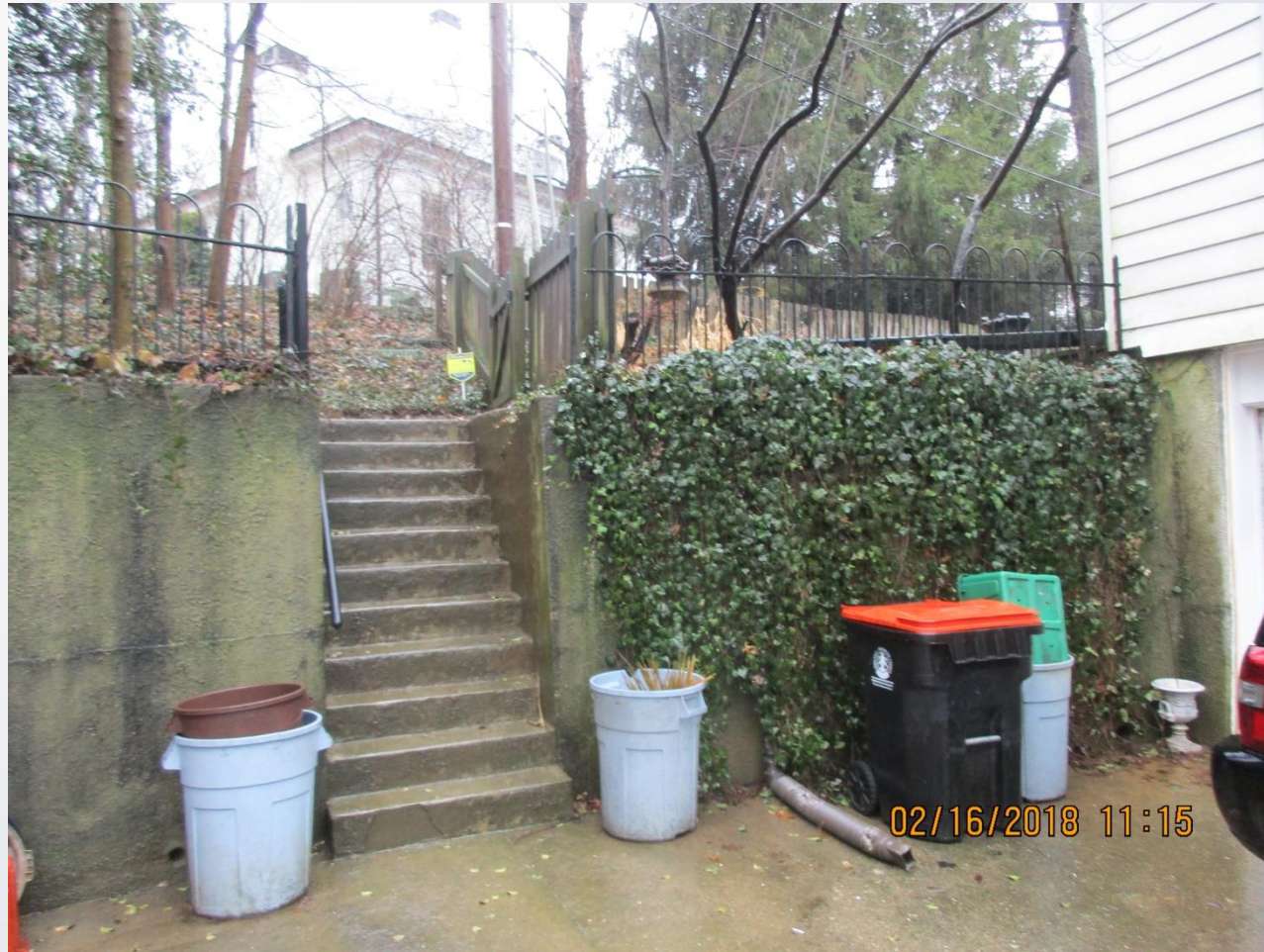
Stairs to Private Yard Area
