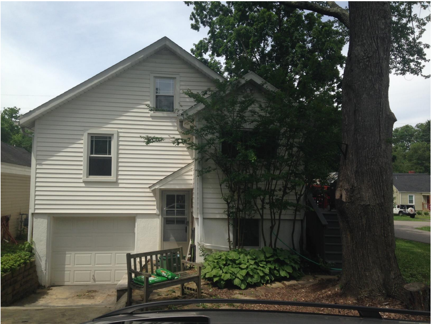
The rear of the existing structure with attached garage to be removed.
