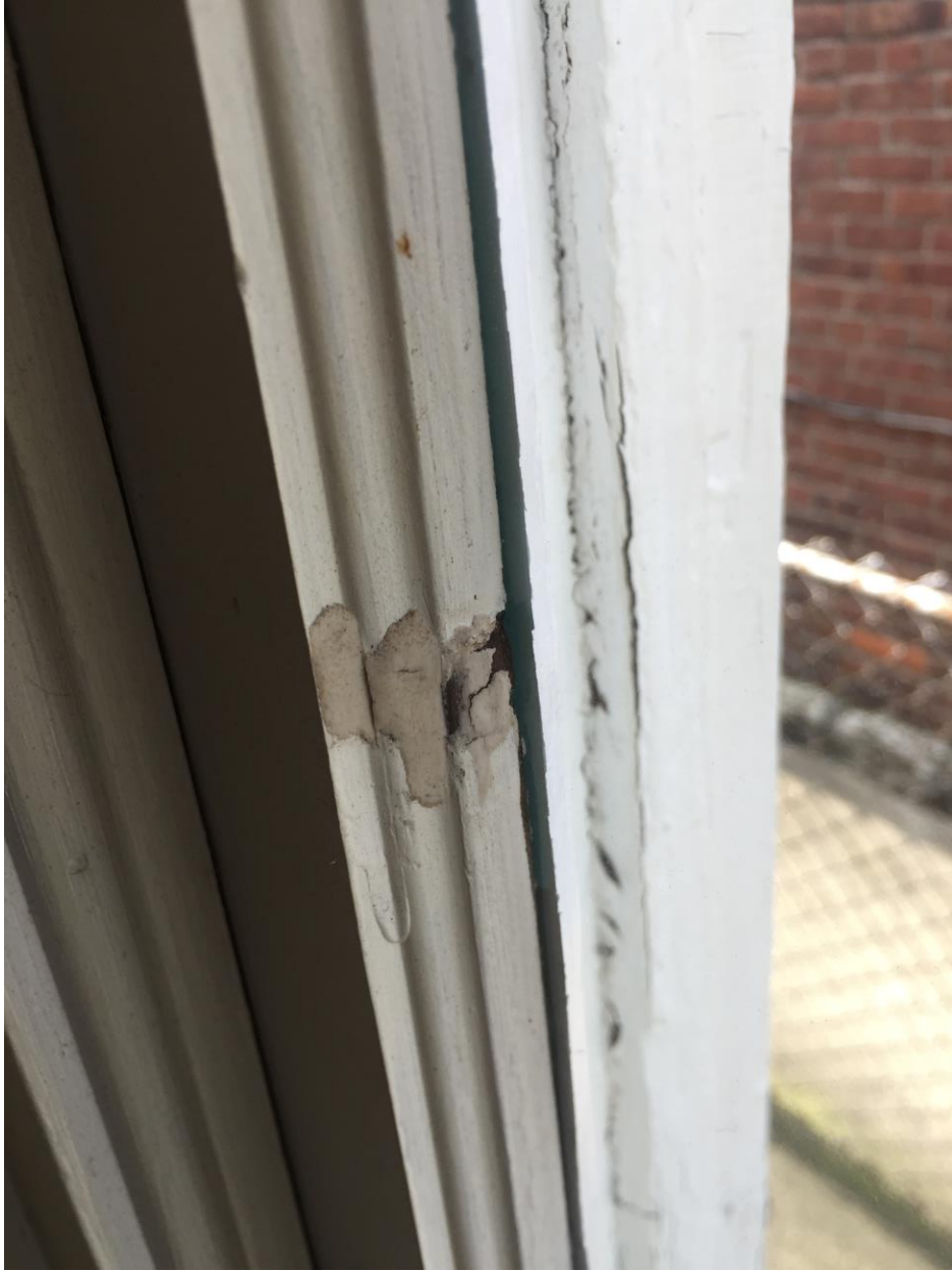
West elevation window #2- class 2
