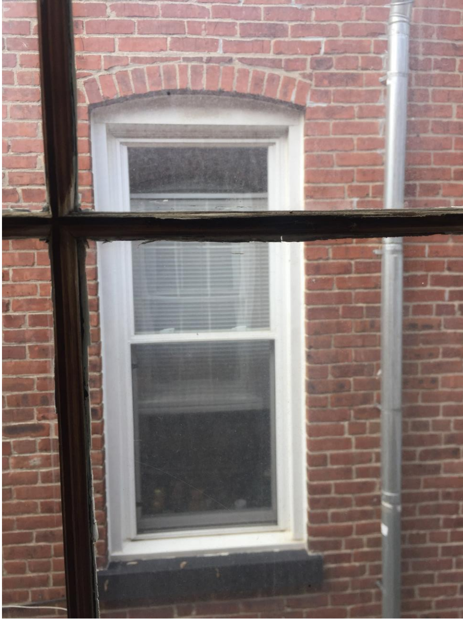
West elevation window #5- class 4
