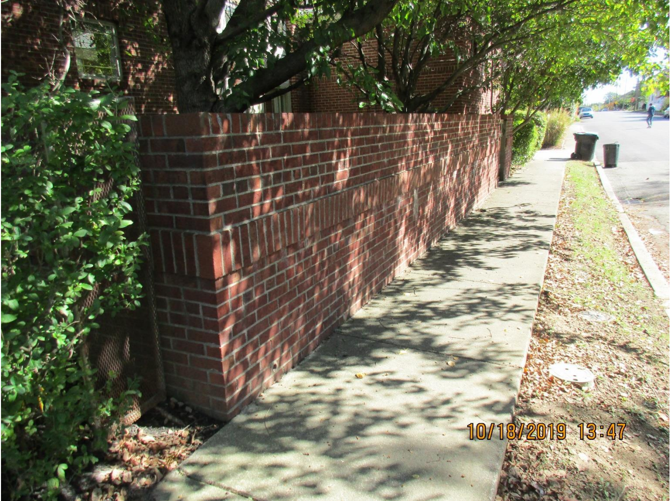
Existing fence on subject property from Dorothy Avenue.
