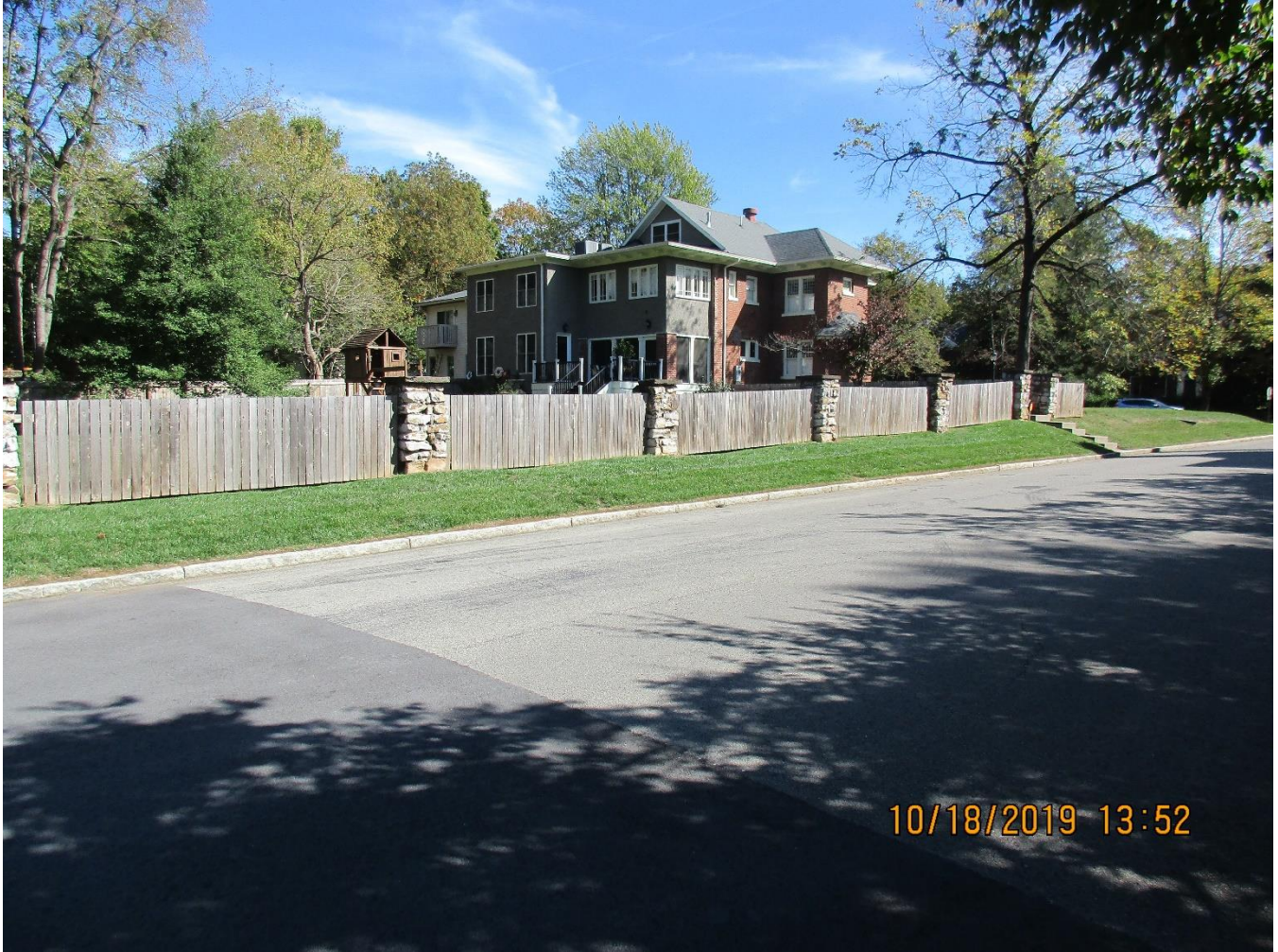
A 54-inch fence in the street side setback at the corner of Douglass Boulevard and Eleanor Avenue.
