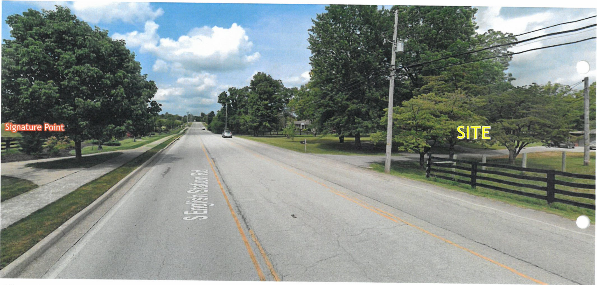
View of S. English Station Road looking north. Site is to the right.
