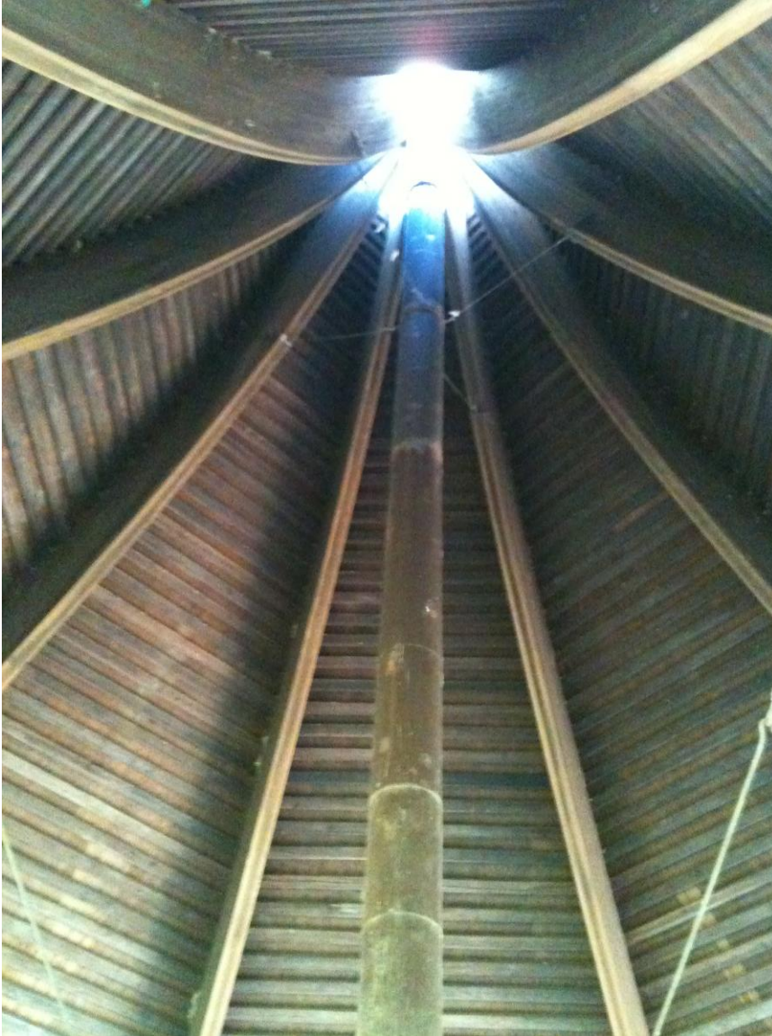
Smokestack with interior roof detail
