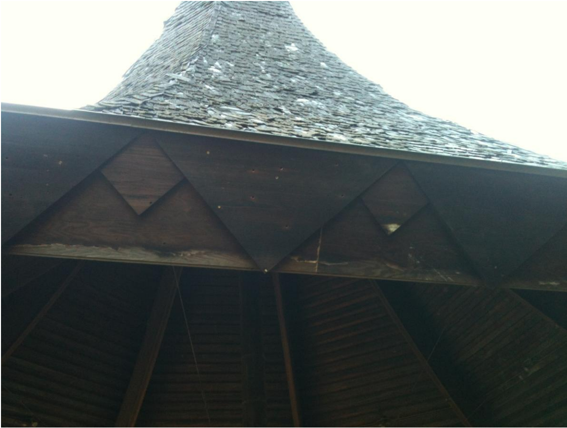
Detail of fascia board dentil pattern
