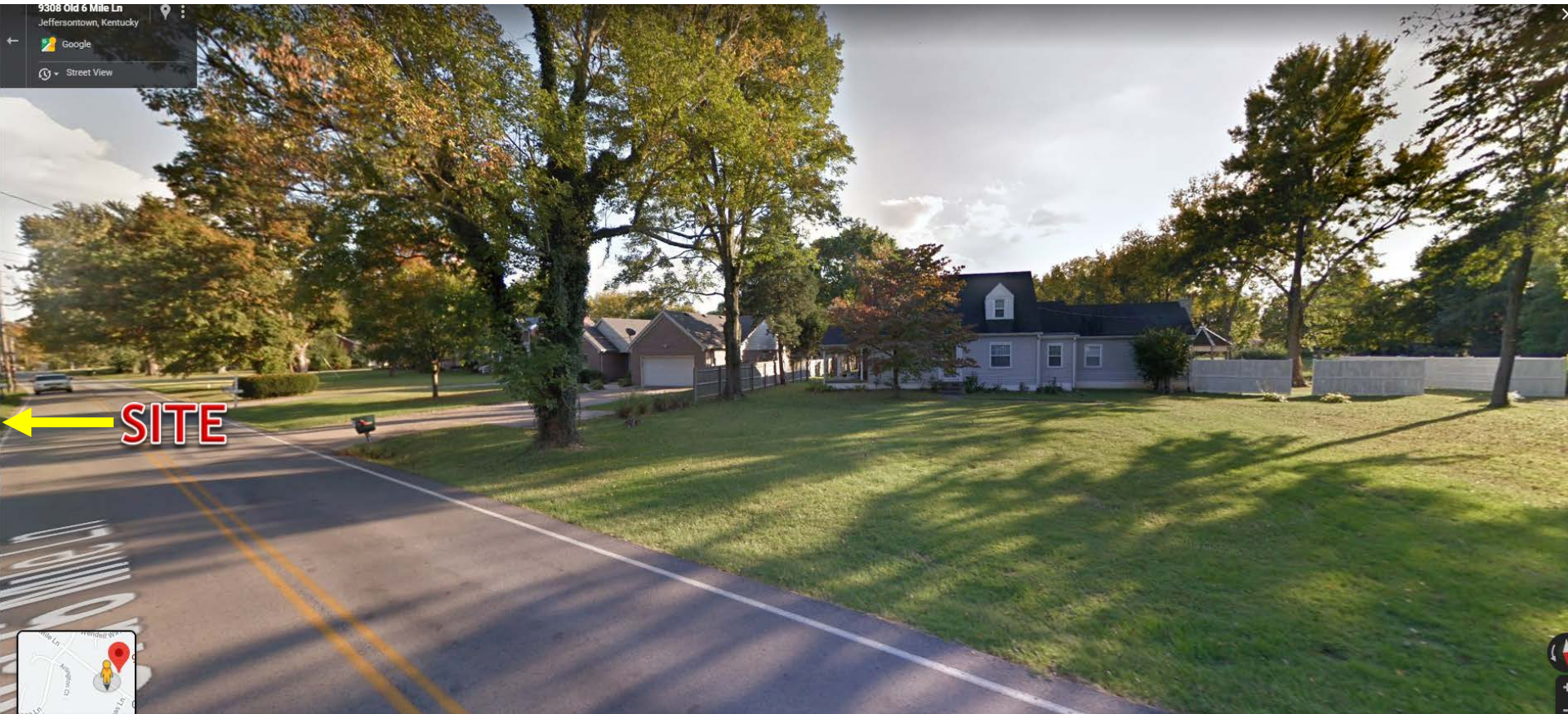
Looking southeast at residences across Old Six Mile Ln from site
