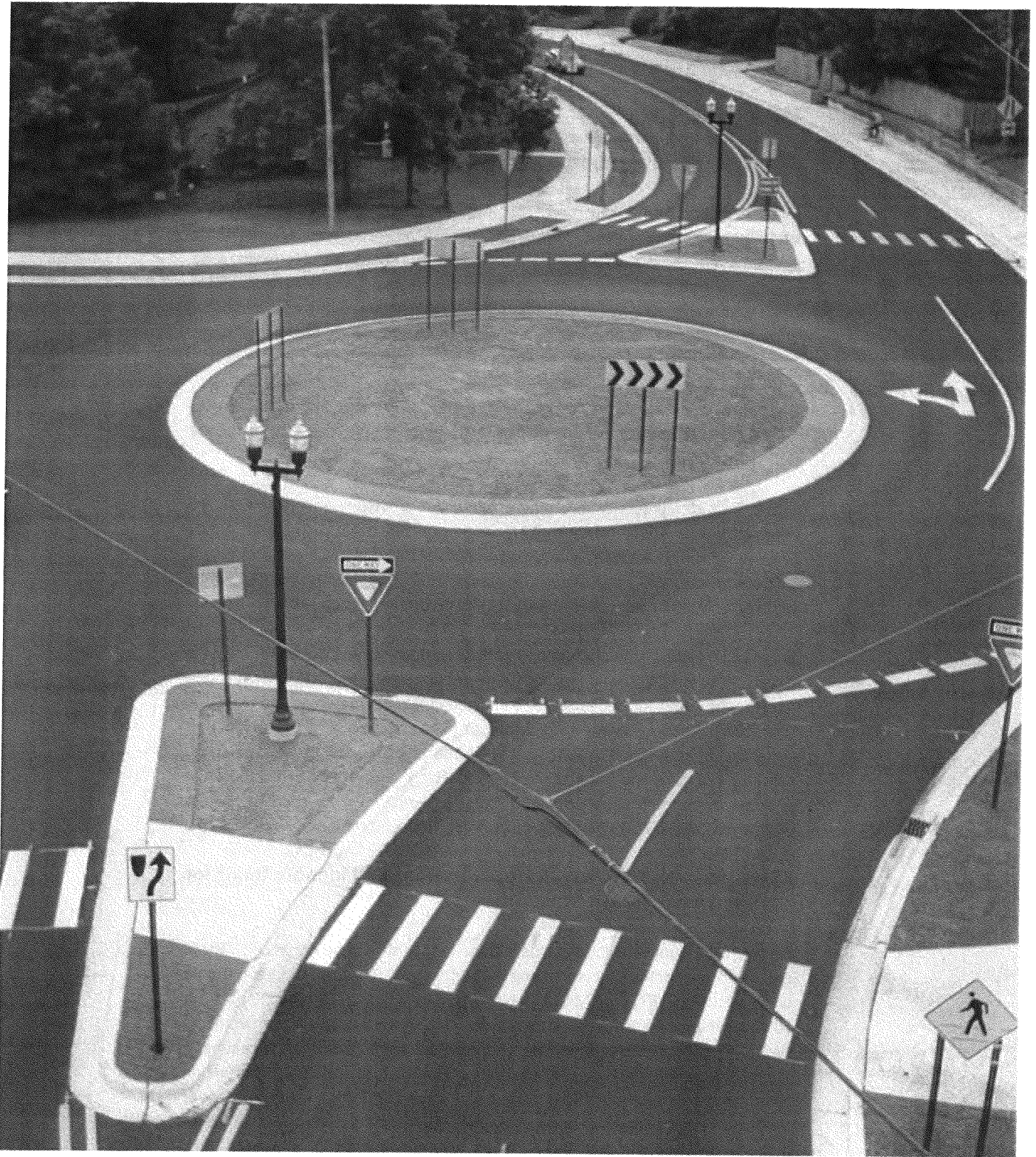
Figure 3.0 - The photo above represents a roundabout in a suburban setting that allows smooth traffic flow and clear pedestrian connectivity in Okemos, Michigan.
