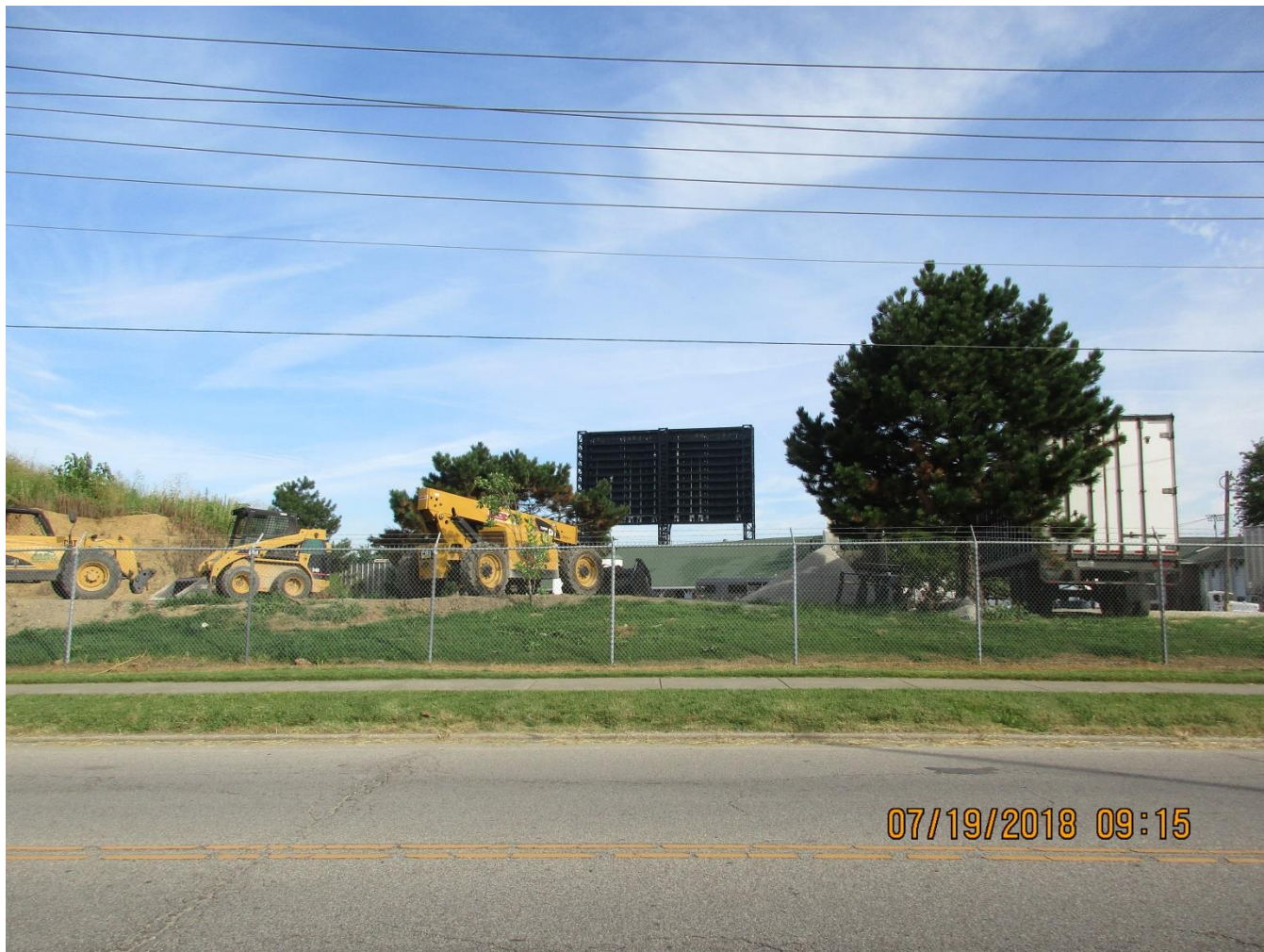
The rear of the existing video board.
