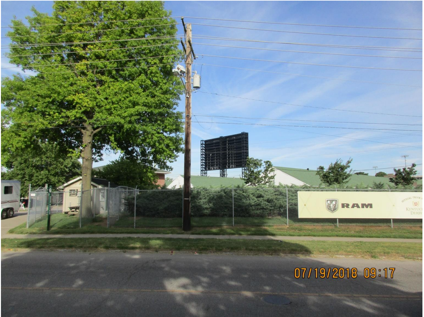
The rear of the existing video board.
