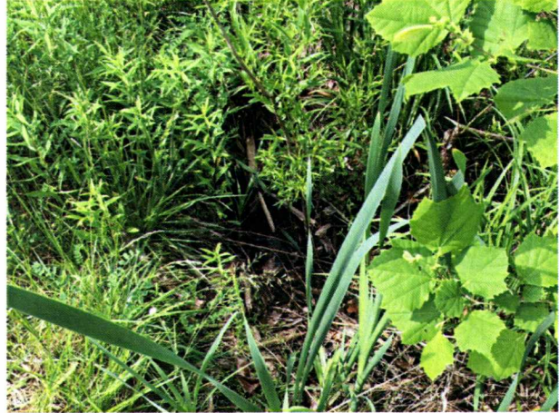
Apparent drain pipe observed in Area 1.
