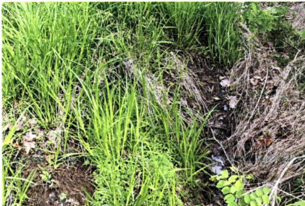
Minor erosion near apparent spring in Area 1
