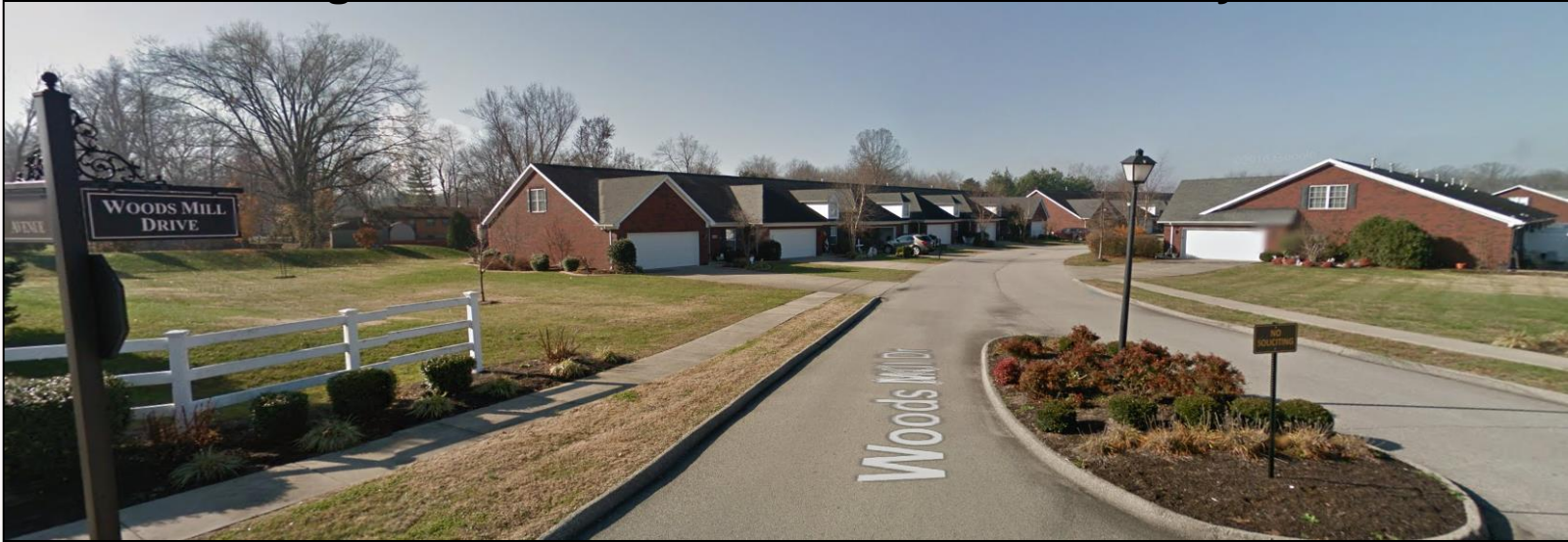
Existing Units on Woods Mill Drive from Tierney Avenue
