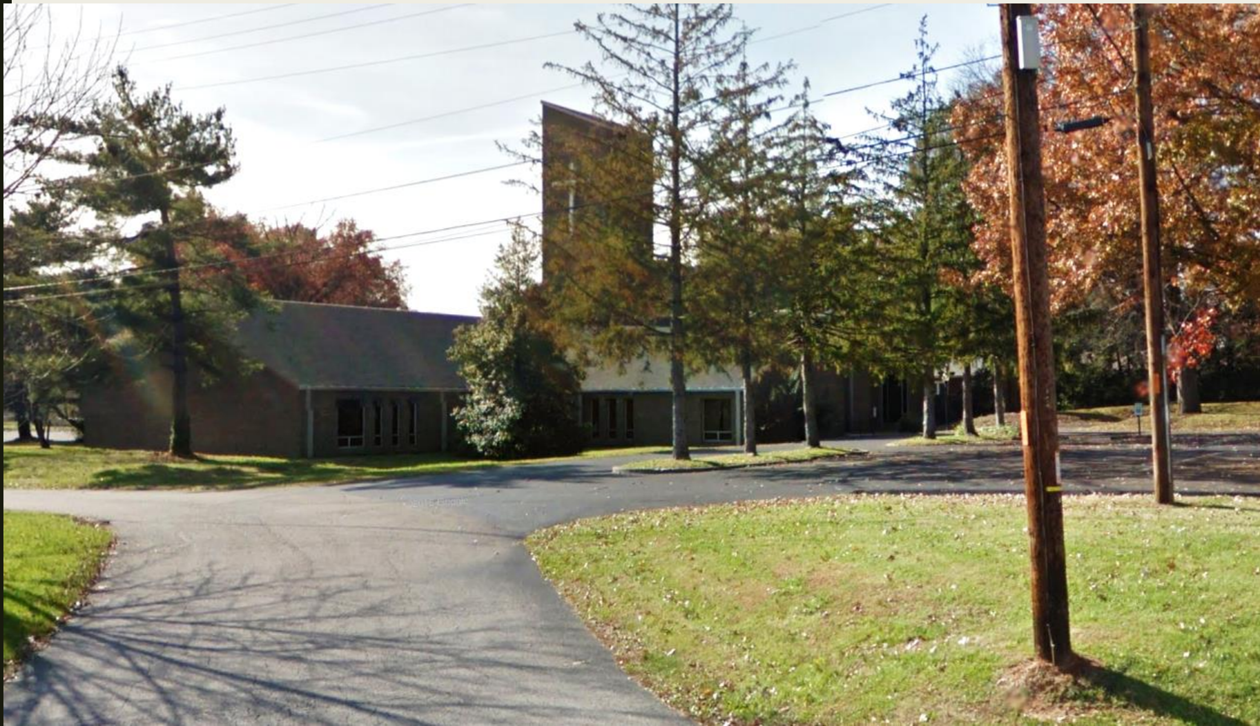
Existing Lifepoint Church, proposed for athletic office and locker room facility.
