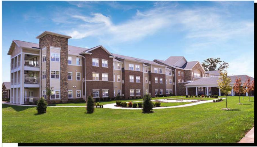
Concept Building ASSITED CARE FACILITY
