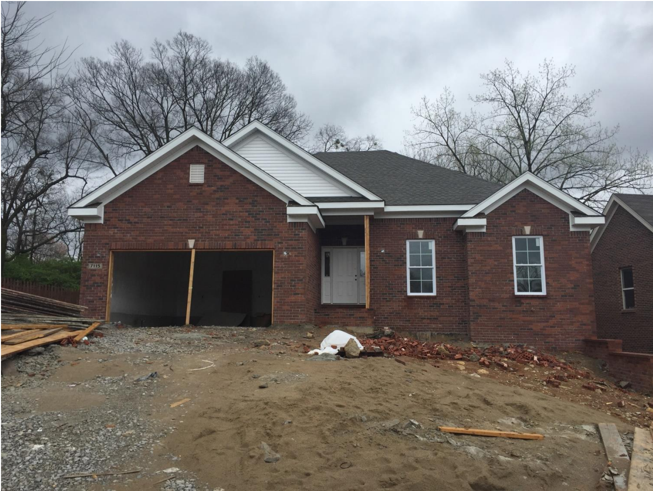
The front of the house under construction.
