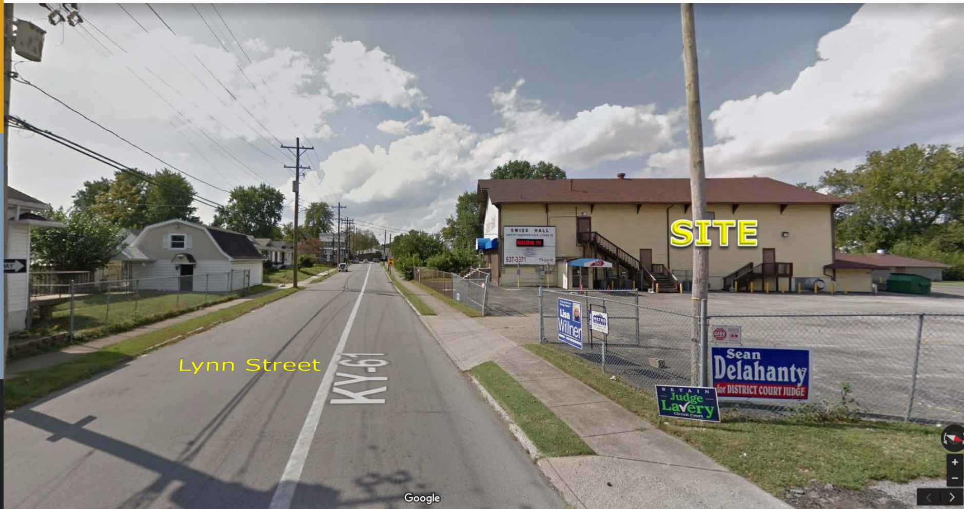
View of Lynn Street, looking west towards Preston Street. Site is to the right.
