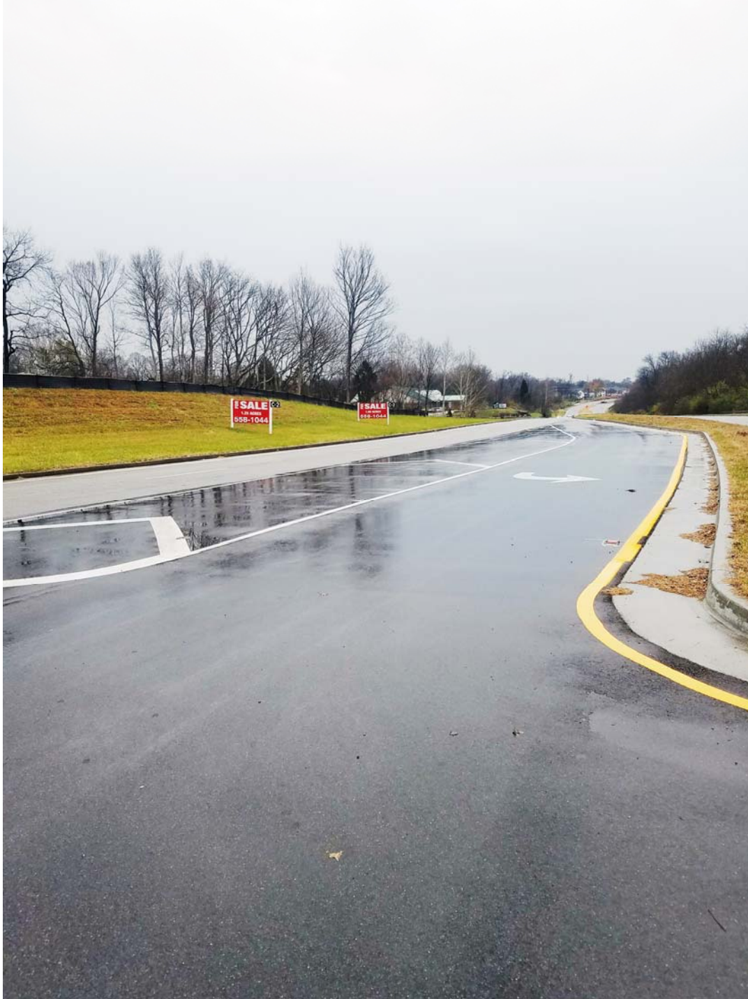
View of full median cut and deceleration lane recently constructed on S. Hurstbourne Parkway looking south. Site is to the right.
