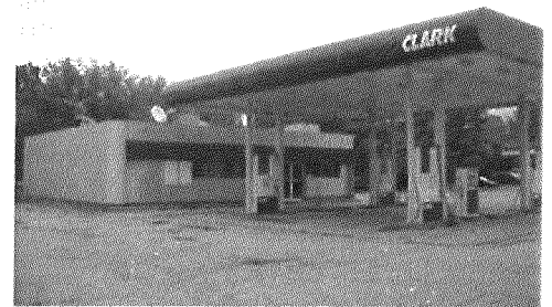
JEFFERSON COUNTY PROPERTY VALUATION ADMINISTRATOR A Louisville developer wants to remodel this building on Bardstown Road and possibly attract a retailer for the space.
