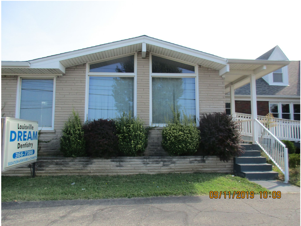
Front of subject property, facing Preston Hwy.
