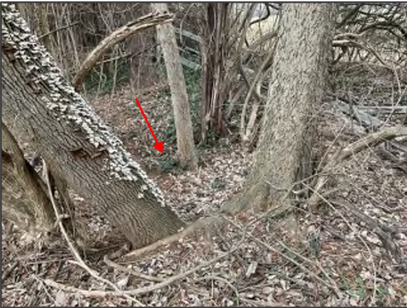
PHOTO NO. 4: Shallow sinkhole with throat (Feature 4)
