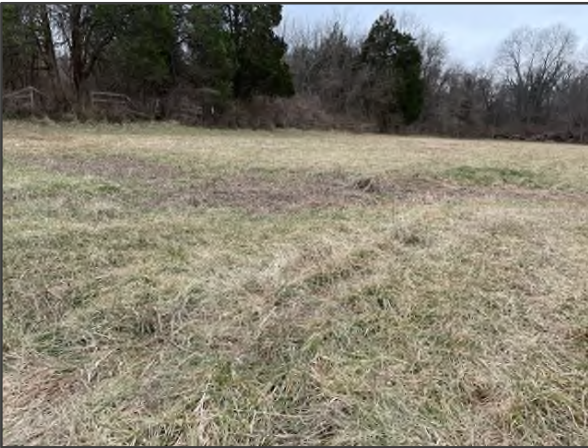
PHOTO NO. 6: Ground subsidence (Features 5 and 6)
