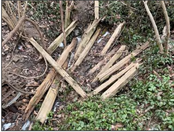
PHOTO NO. 9: Sinkhole at southwest corner (Feature 7)
