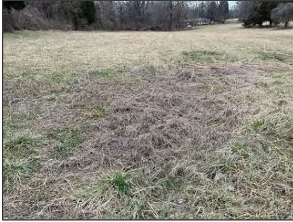
PHOTO NO. 7: Ground subsidence/differing vegetation (Feature 5)
