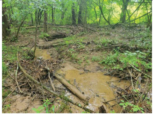
Photo 12: Standing water observed in drainage swale – downslope portion of (AOI-2).
