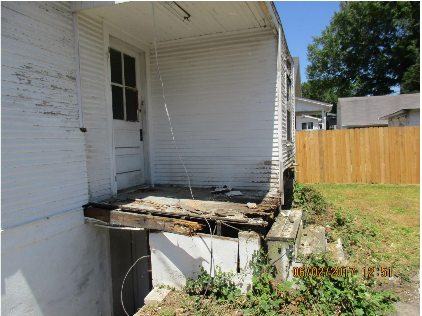
The existing dilapidated addition to be removed. The new addition will be constructed in this approximate location, with a deck beside it.
