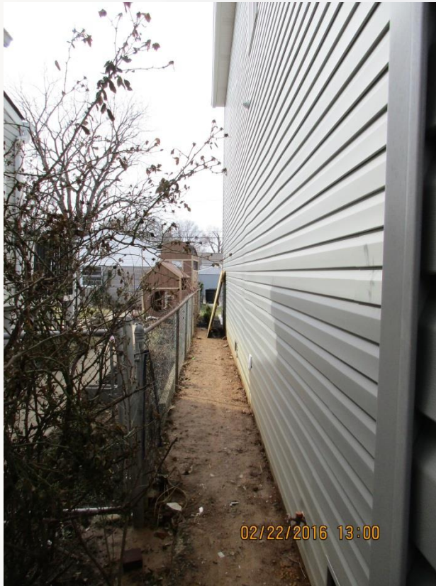
Looking Southwest along the southern side of the property at the setback from the neighbor's fence line.
