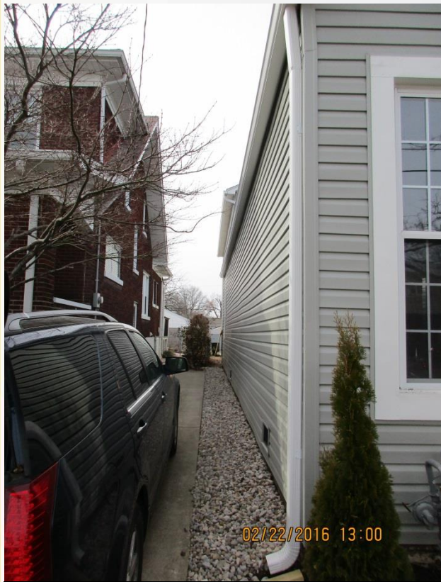
Looking Southwest along the southern side of the property from the front.
