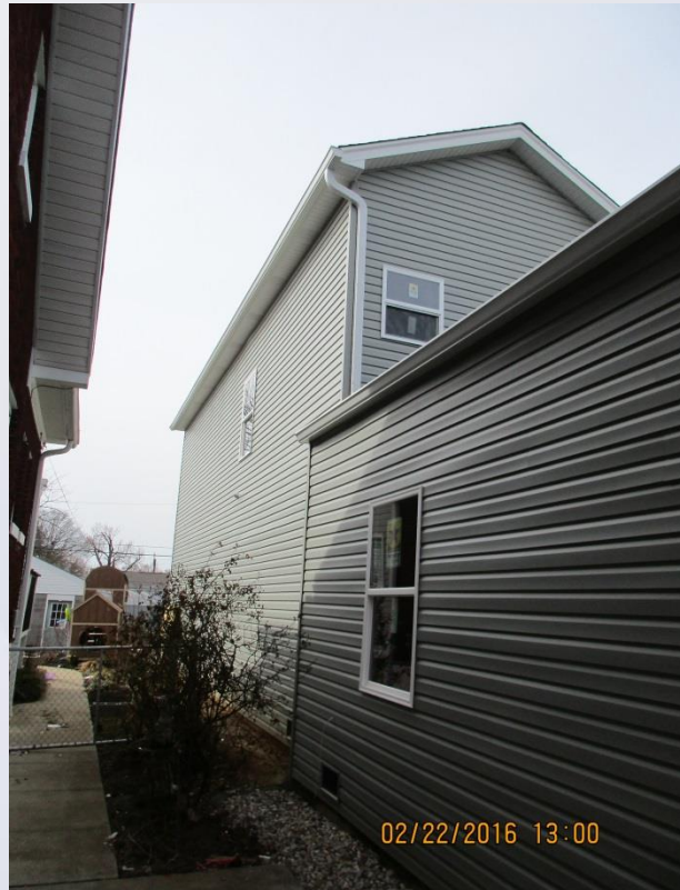
Looking Southwest along the southern side of the property at the two story rear addition.
