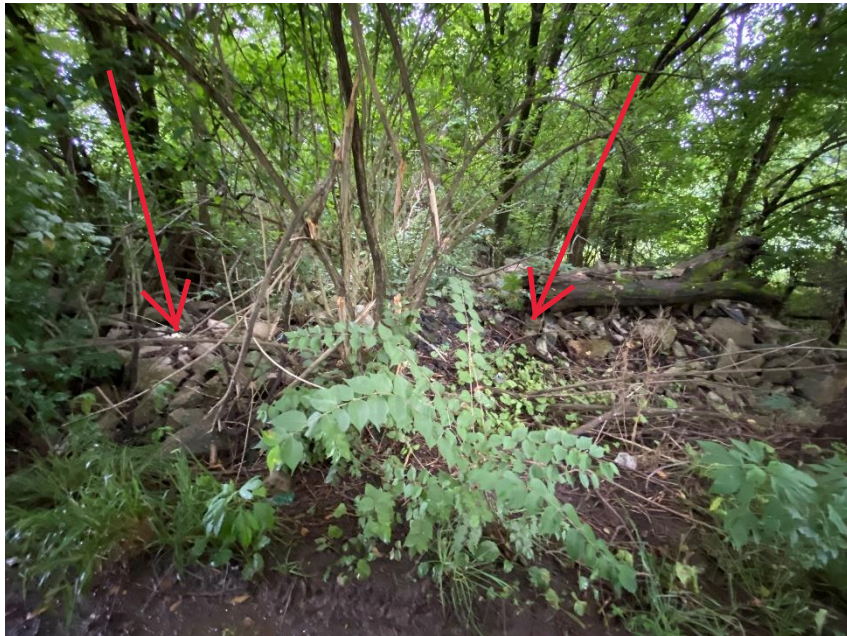
View of possible sinkhole filled in with rock and debris approximately 20'x8' in size. (N 38.106582° W 085.680512°)
