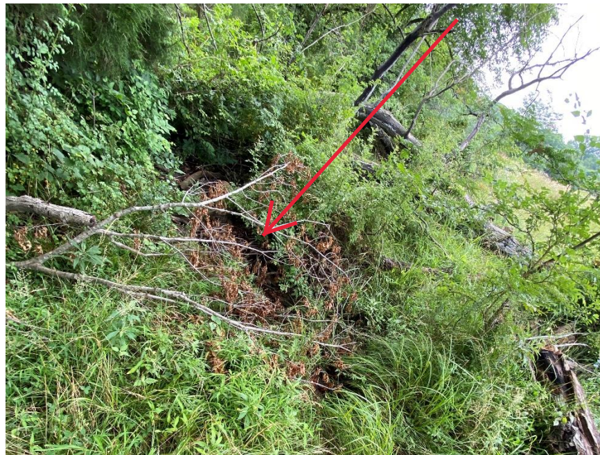
View of possible sinkhole filled with rocks and tree limbs (N 38.108676° W 085.684726°)
