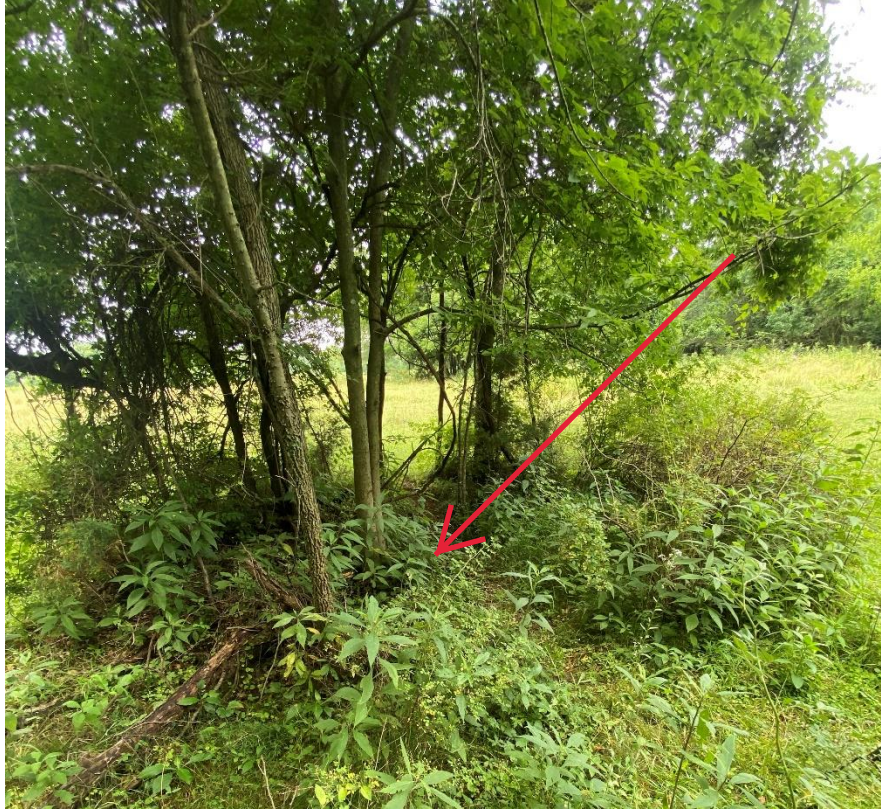
View of possible sinkhole surrounded by small trees 6x'6 in size (N 38.108423° W 085.683031° )
