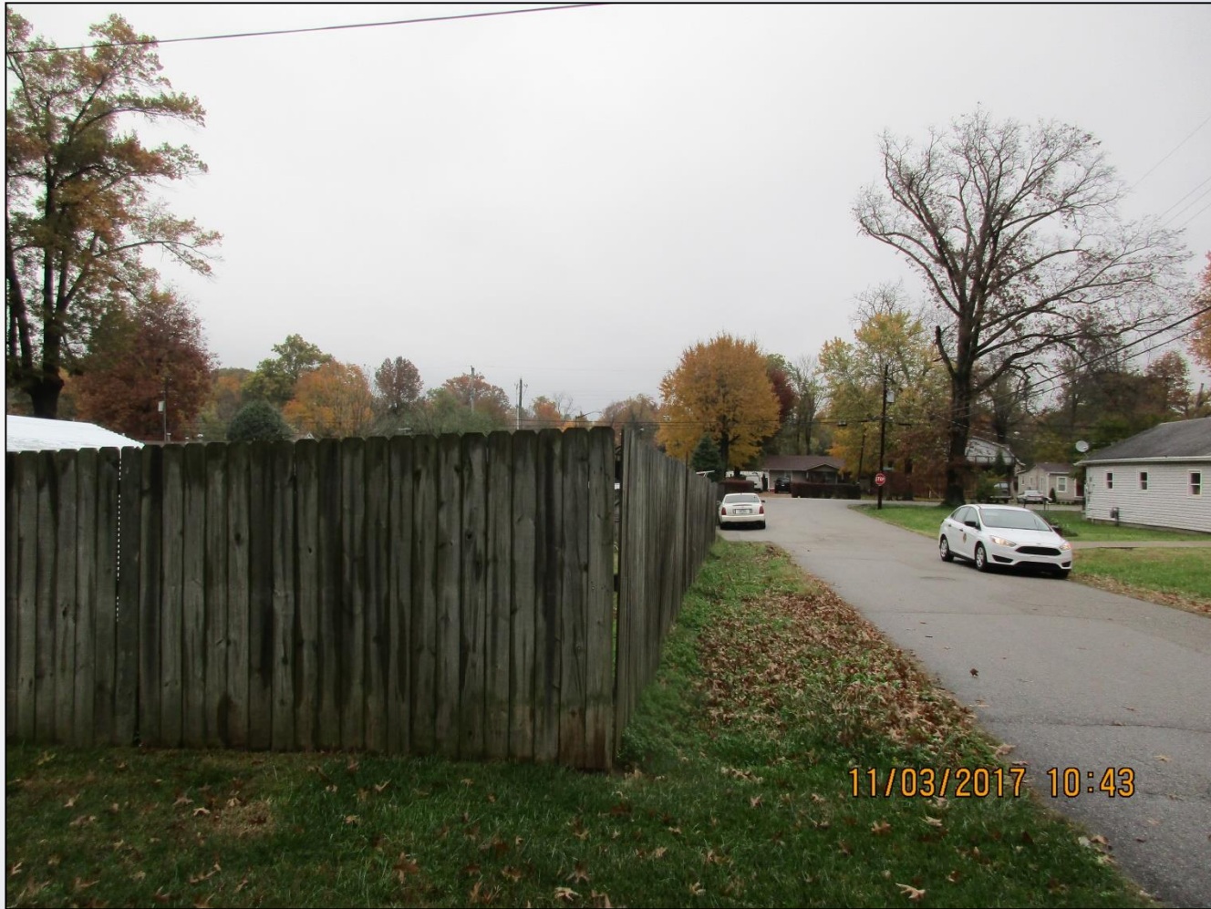
The southern section of fence.
