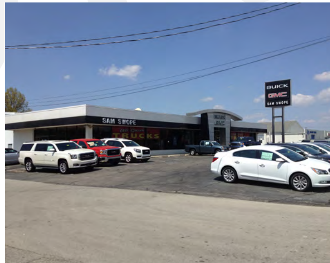
Large tracts have been devoted to auto sales, with parking fields for auto display in front of building.
