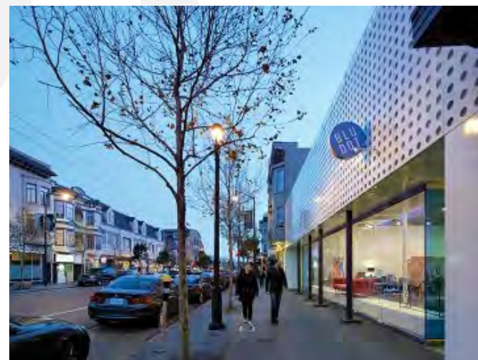
Parapet walls create the illusion of second story on this simple but elegant commercial building.
